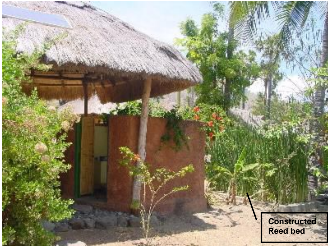
Figure 6-2 Atauro Island greywater treatment system.
